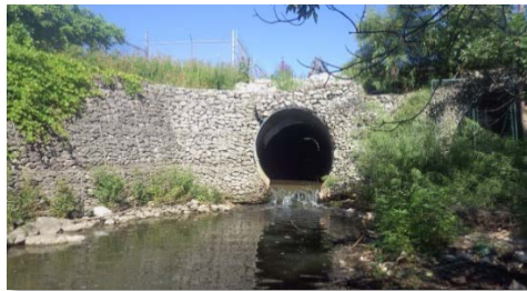
The Stormwater Asset Management Plan includes managing the City's storm sewer network effectively and efficiently
