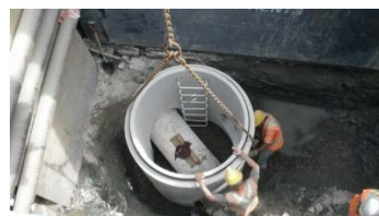
Installation of storm pipe infrastructure
