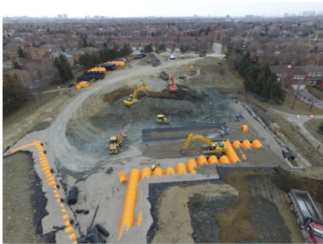
Installation of storage chambers at Eastgate Park
