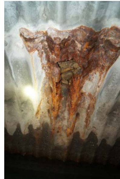
Corroded metal storm sewers require replacement
