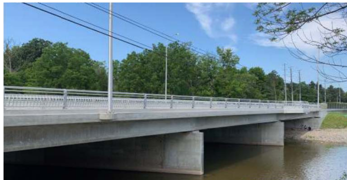
Completion of the Creditview Road bridge renewal – includes a new cycling platform on the west side of the bridge
