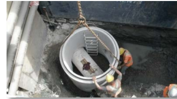
Installation of storm pipe infrastructure
