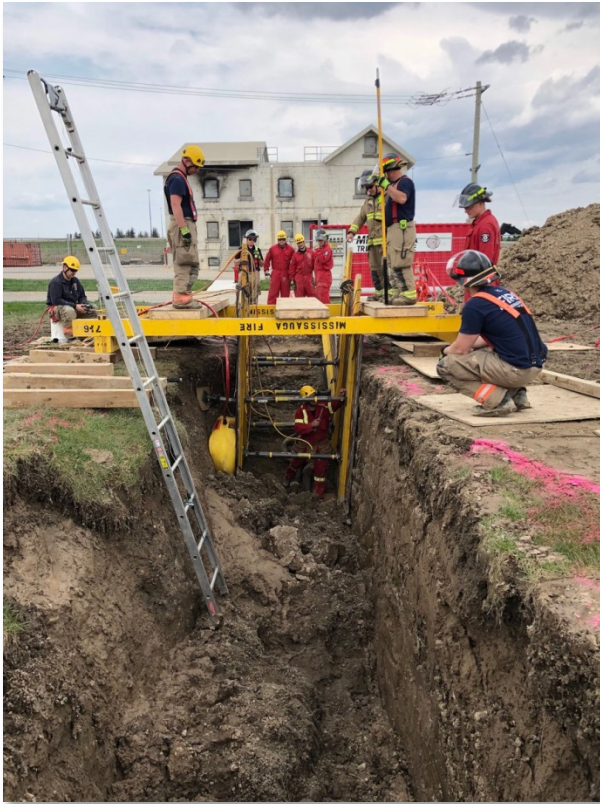
Live Trench Rescue Training at Garry W. Morden Centre
