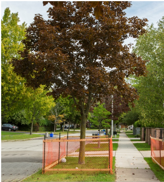
Protective Hoarding around City Tree
