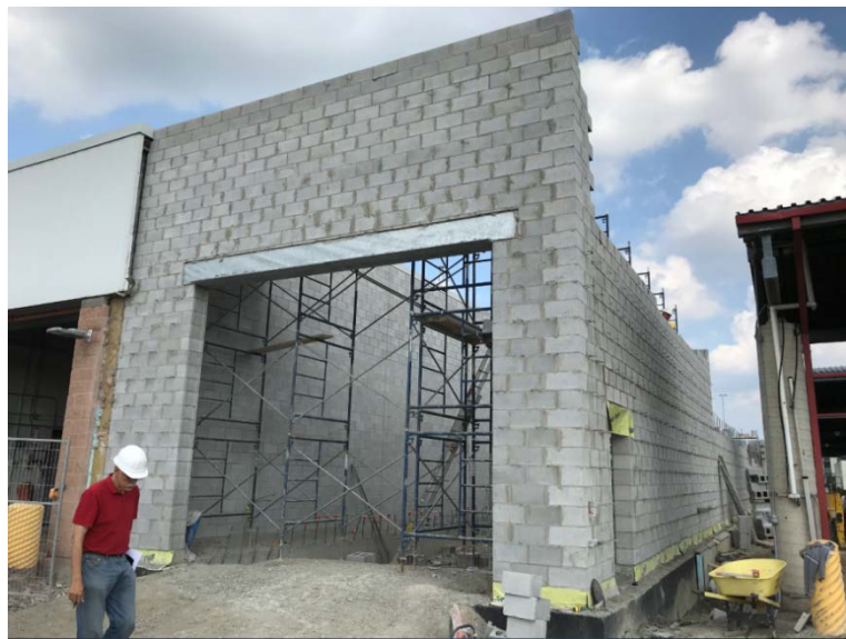
Malton Satellite Terminal – Wash Bay Addition
