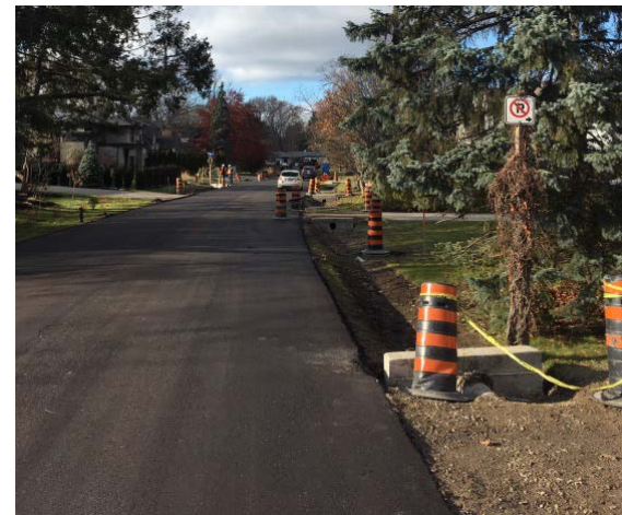
Ditch Regrading on Old River Road
