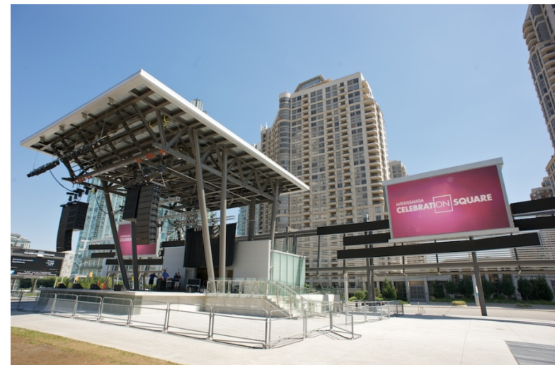
Celebration Square stage and digital signs: location is also a Wi-Fi hot-spot
