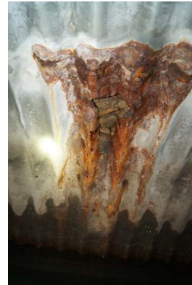
Corroded metal storm sewers require replacement
