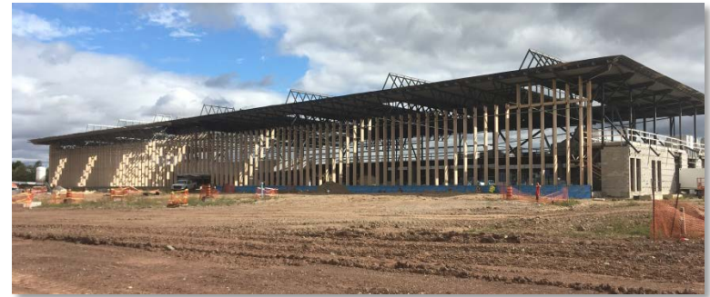
The Churchill Meadows Community Centre will be the 12 th community centre in the city. It is shown here under construction
