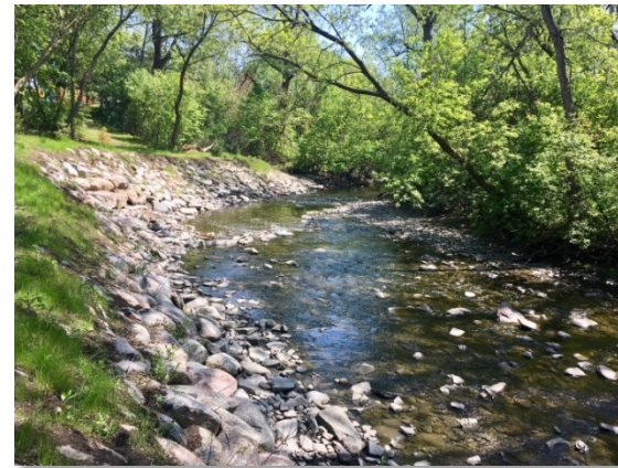
Erosion control projects improve the condition of the City's watercourses
