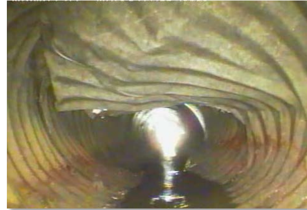
Renewal of storm sewers is a major focus of the Business Plan
