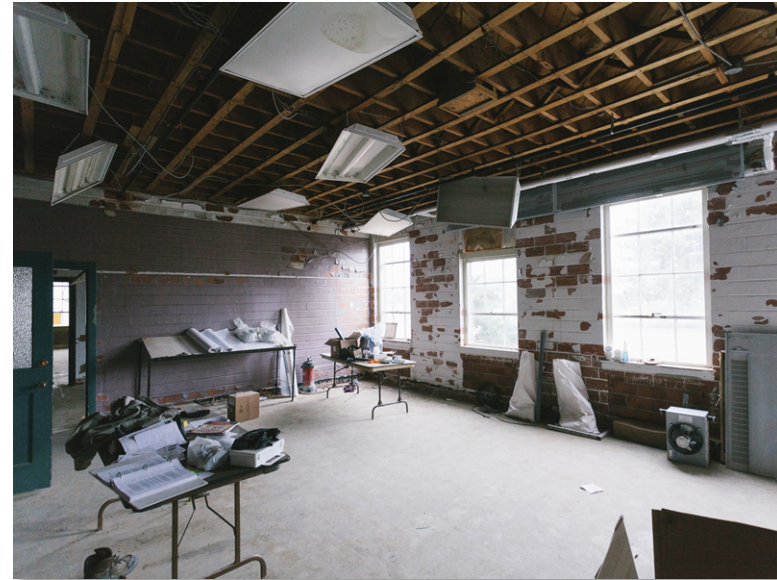
An unfinished room at the Small Arms Inspection Building
