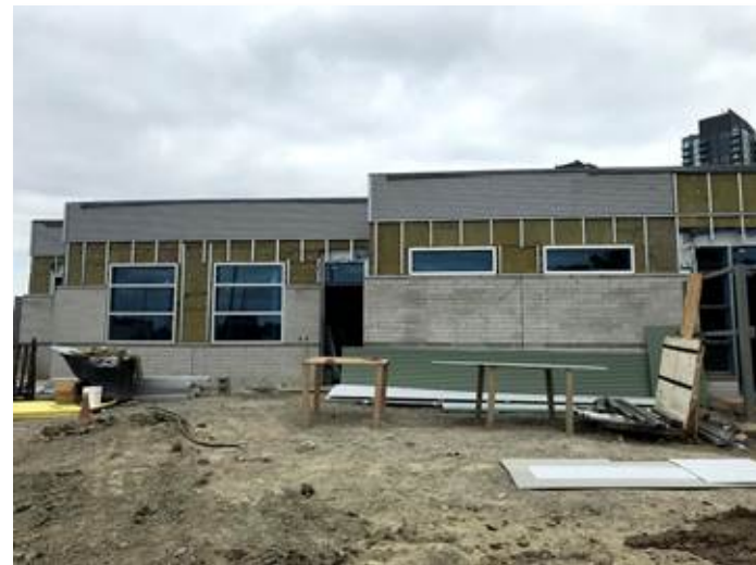
New Fire Station 120 Construction
