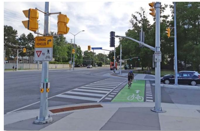
Completion of bicycle crossrides on Burnhamthorpe Road
