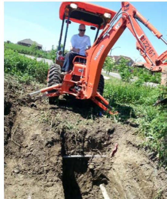
Park Operations staff working on irrigation repairs
