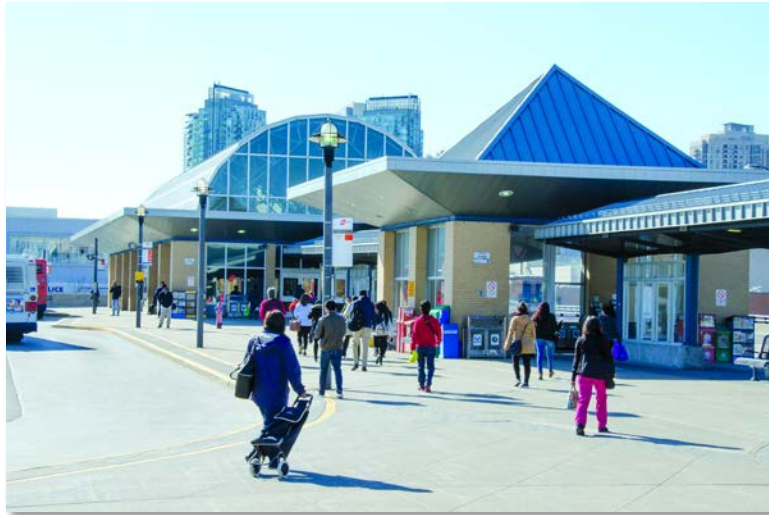
City Centre Transit Terminal
