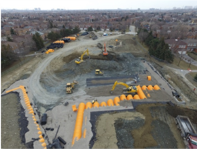
Installation of storage chambers at Eastgate Park
