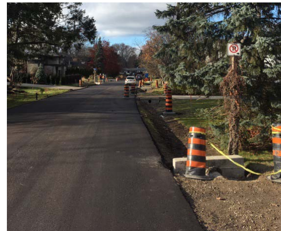
Ditch Regrading on Old River Road
