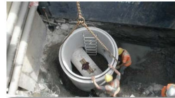
Installation of storm pipe infrastructure
