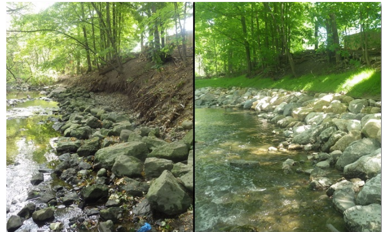
Little Etobicoke Creek photographed in 2016 (left) Completed erosion control project (right)
